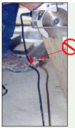
This cord has been spliced using a wire nut. Spliced cords are very dangerous!
