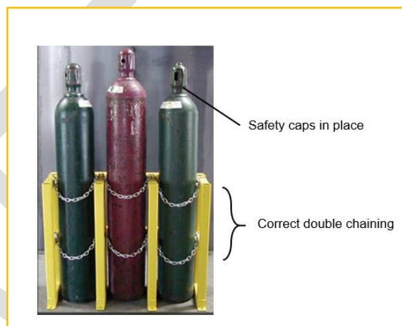
Figure 6-1: Image of gas cylinder storage using the proper two-chain method.
