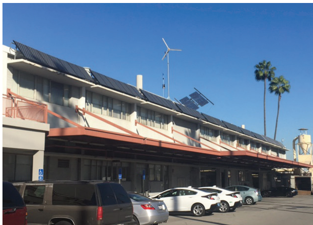
Figure 9: Solar Panels and Wind Turbine on E&T
