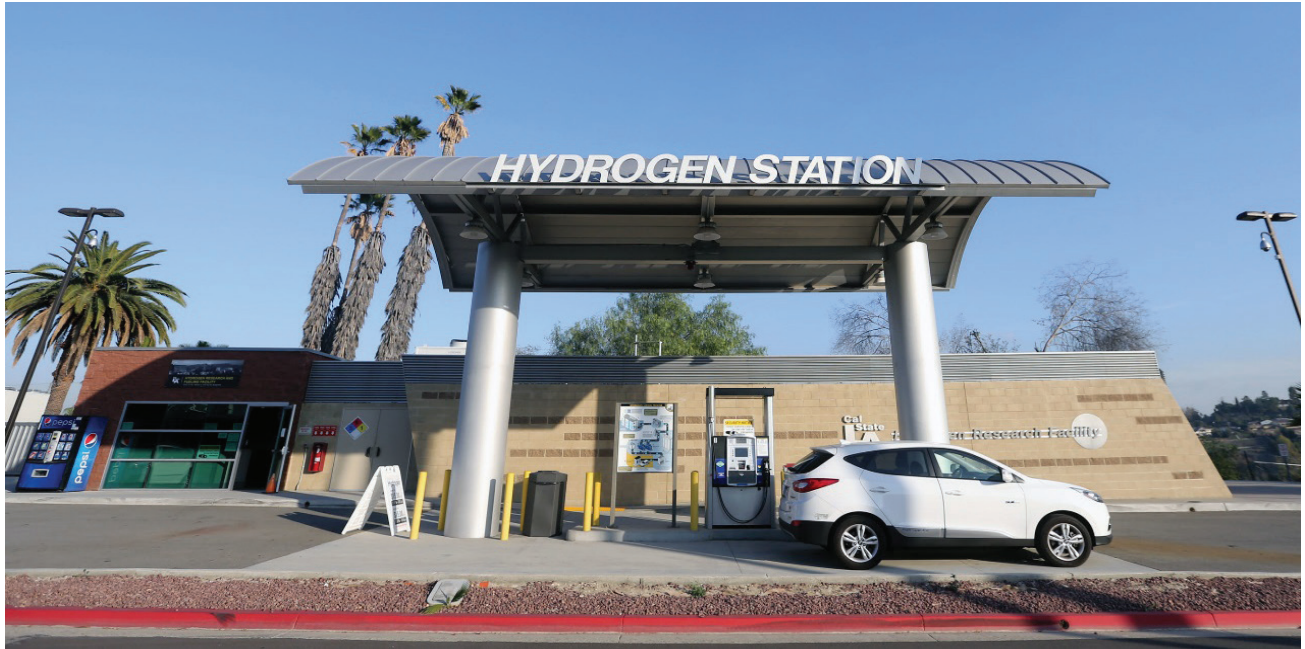
Figure 22: Cal State LA Hydrogen Station
