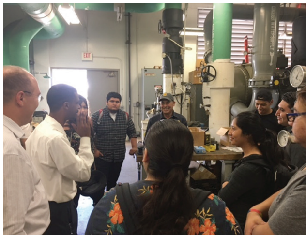
Figure 21: CALL Tour of Cal State LA's Central Plant
